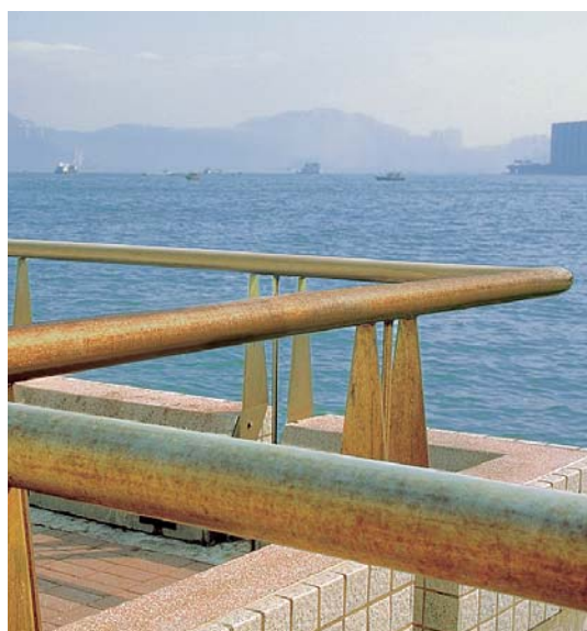
Figure C Seawater splashing or spray will corrode Type 316 stainless steel. The rough surface finish on these railings and infrequent washing made the problem worse. (Photo Courtesy of the Nickel Institute)
