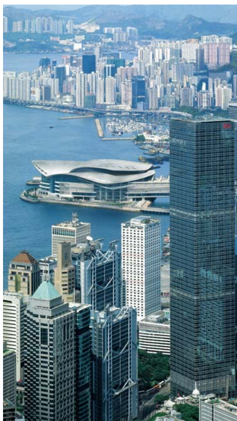
Figure A and B Cheung Kong Center is the high-rise building in the foreground of Figure A. The entrance and other details are visible in Figure B. Type 316 stainless steel with smooth surface finishes was an excellent choice because it is exposed to pollution and coastal salt. Window washing tracks were built into the building for easy cleaning. As shown in Figure A, it is in close proximity to the harbor. (Photos Courtesy of Outokumpu)
